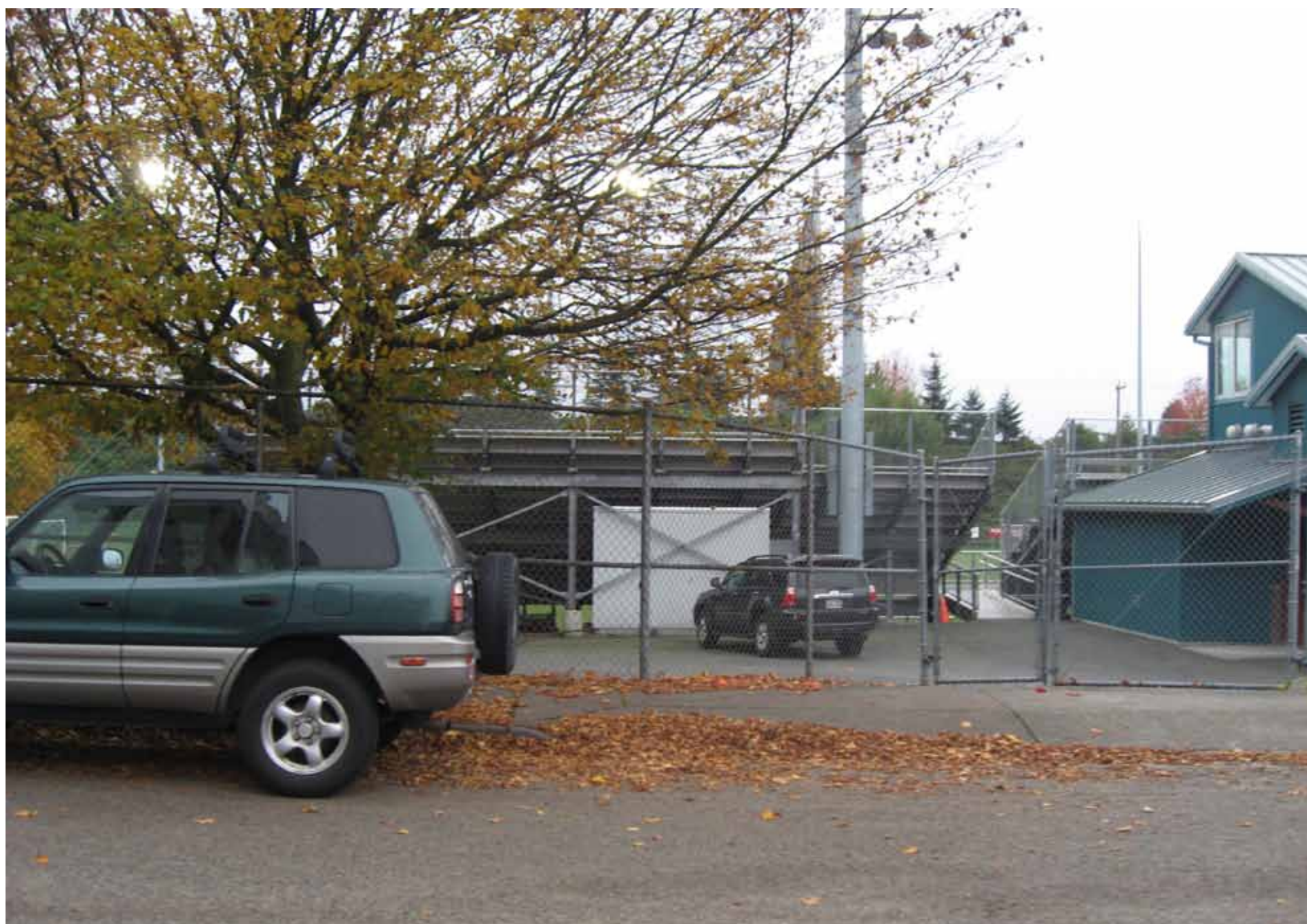
VIEW FROM PROJECT SITE LOOKING SOUTH ACROSS BARRETT
