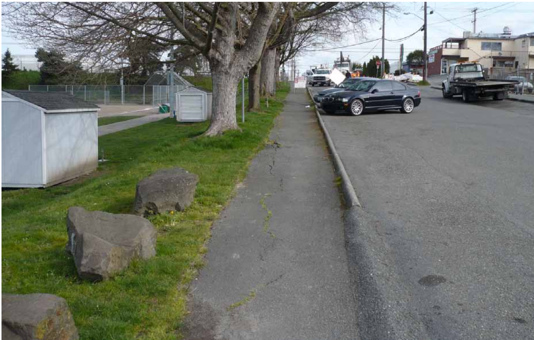
TYPICAL SIDEWALK CONDITION AT 17TH AVE
