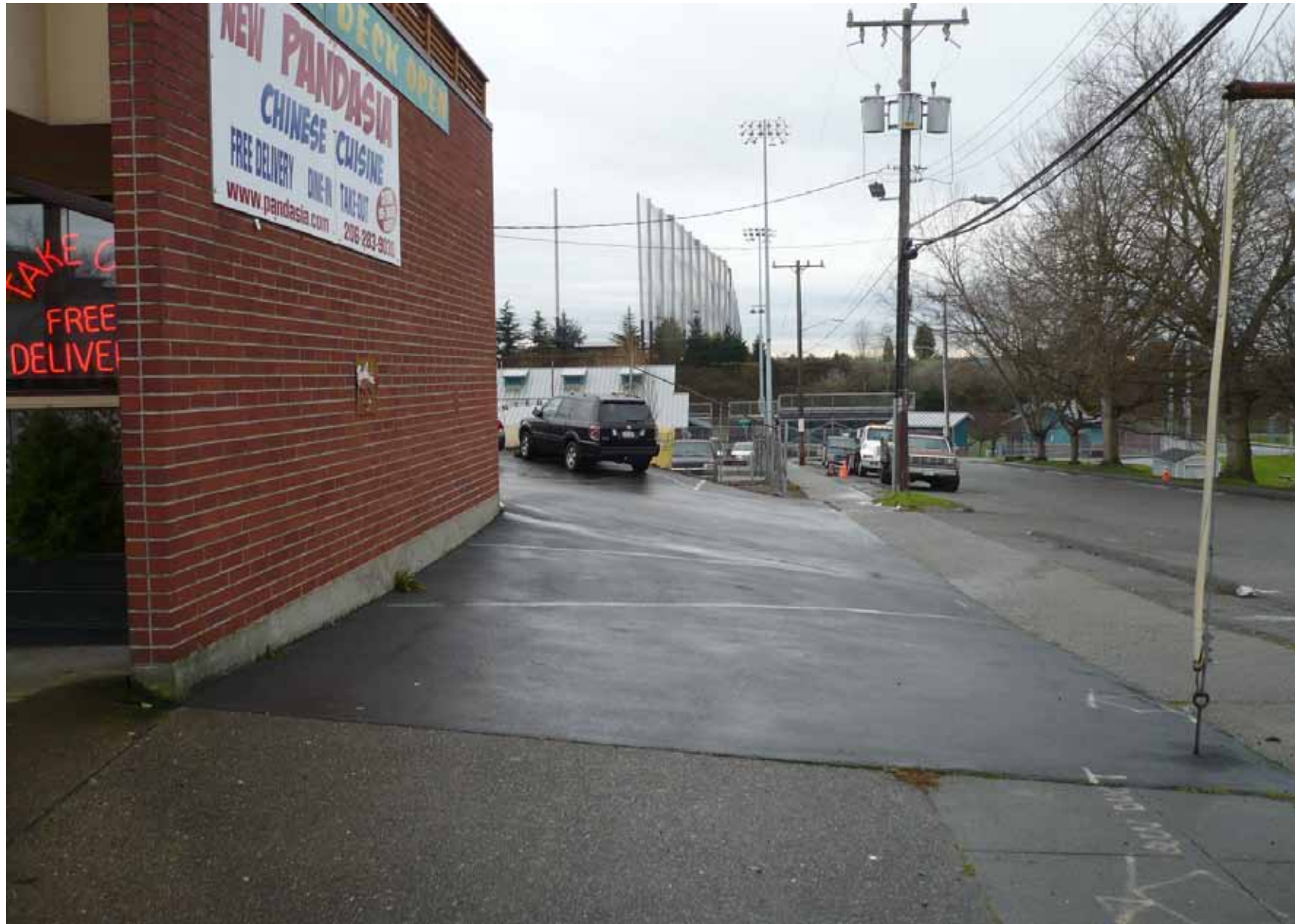
17TH AVE AT PANDASIA. FACE OF BUILDING IS AT PROPERTY LINE
