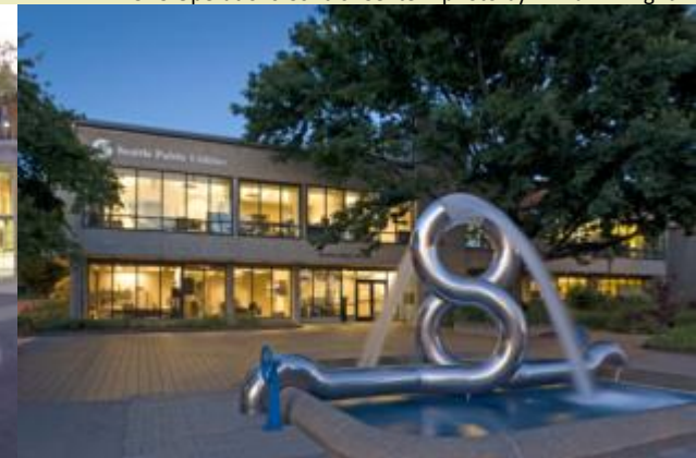
SPU Operations Control Center - photo by William Wright
