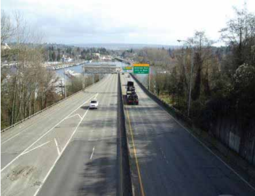
Portage Bay Bridge looking east from Delmar Drive East
