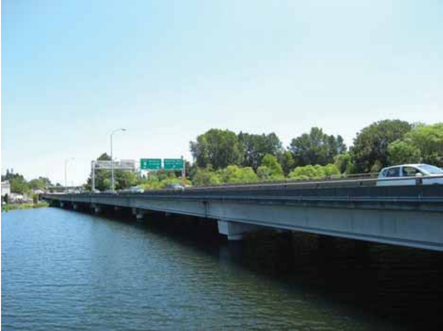
Portage Bay Bridge looking southeast from boat
