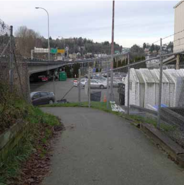
Bill Dawson Trail looking west at westbound on-ramp (NOAA at right)
