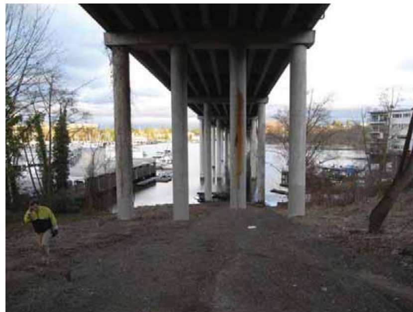
Portage Bay Bridge looking east from Boyer Avenue East
