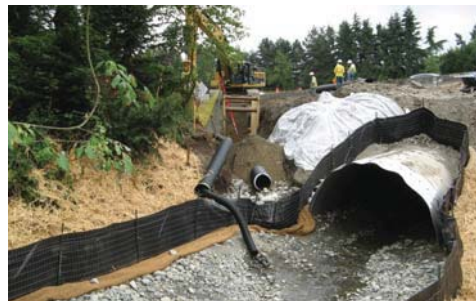
New and wider culverts will provide better fish passage on the Eastside.
