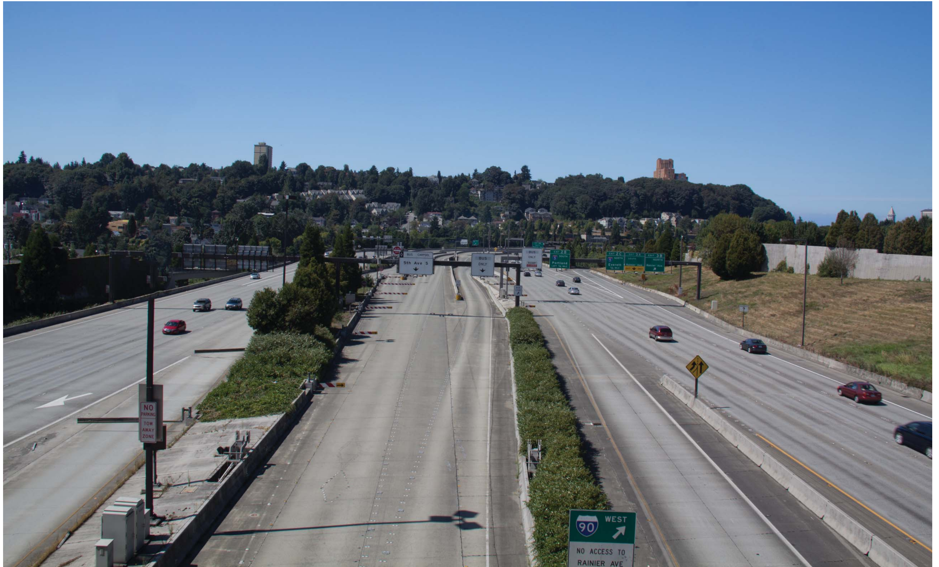
Existing Conditions of I-90 from Mount Baker Tunnel
