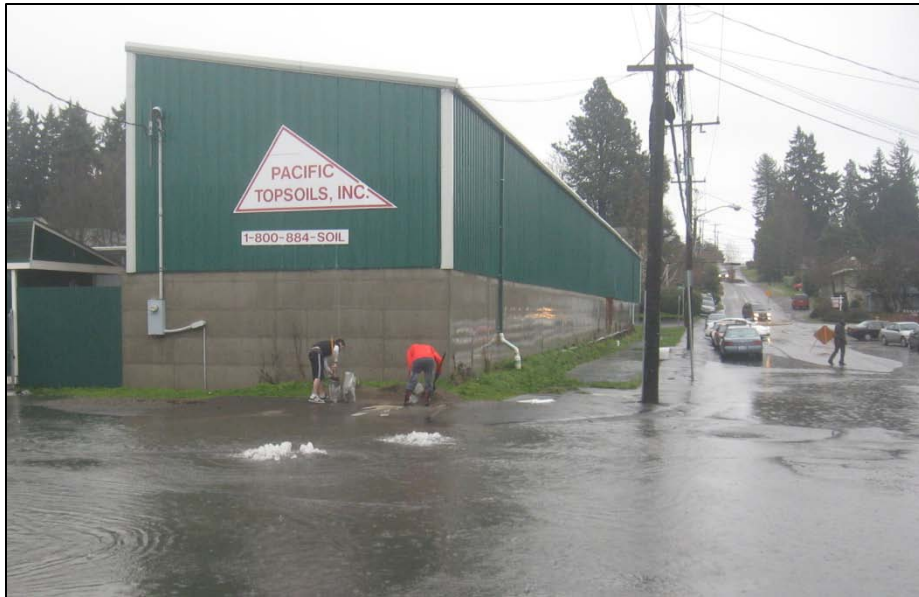
Stormwater surging out of inlets
