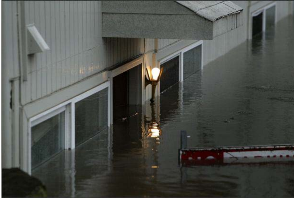
Daylight basement apartments On Midvale south of N 107 th St
