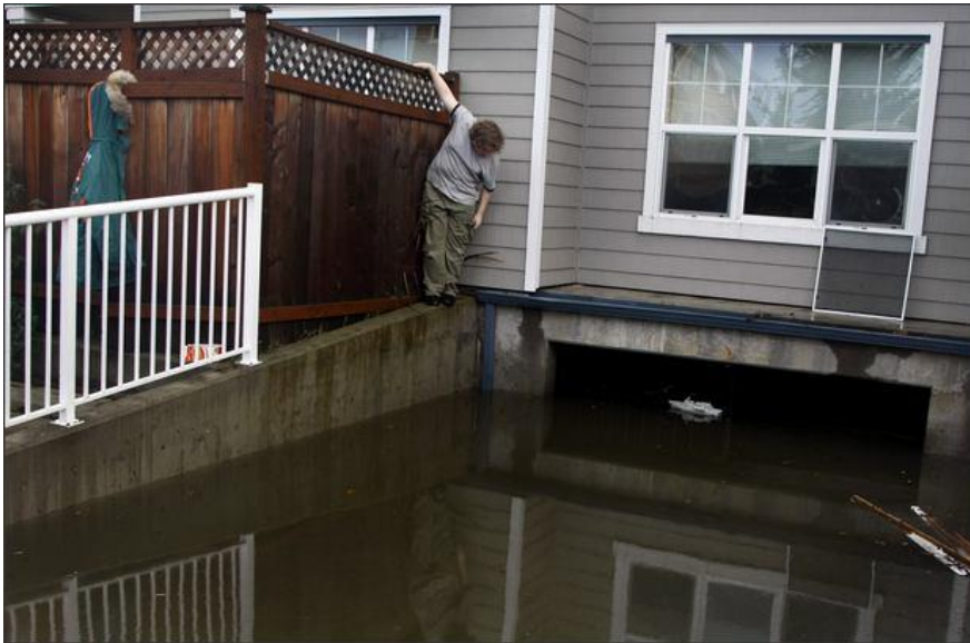
Condo parking garage off alley between Stone & Midvale south of N 107 th St
