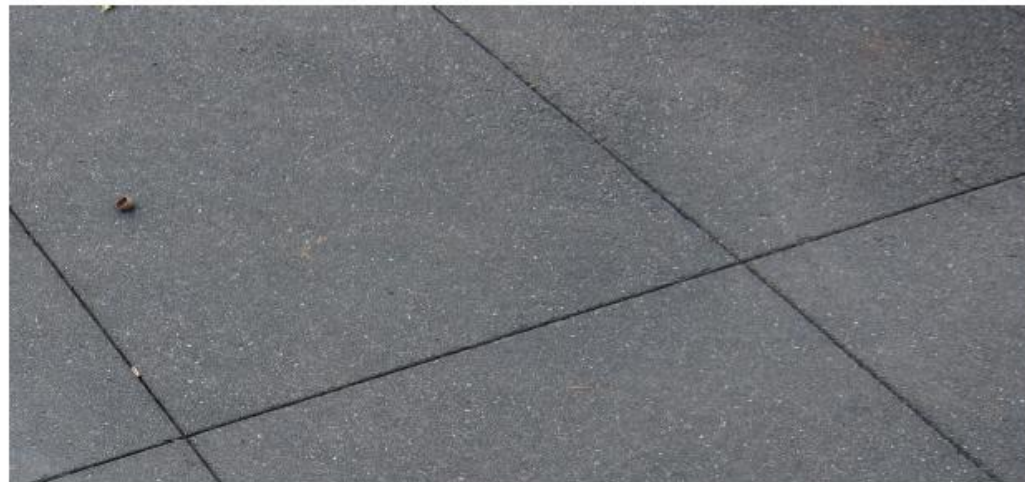
Lithocrete Paving with saw-cut joints
