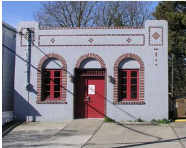
Fire Alarm Sub-Station No. 1 built circa 1921, modernist interpretation of Mediterian or Mission Revival
