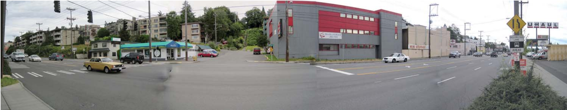
15th Ave West looking across to Fire Station 20 site
