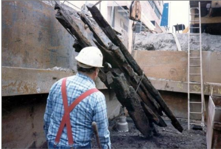
2002 relieving platform repairs (to right)
