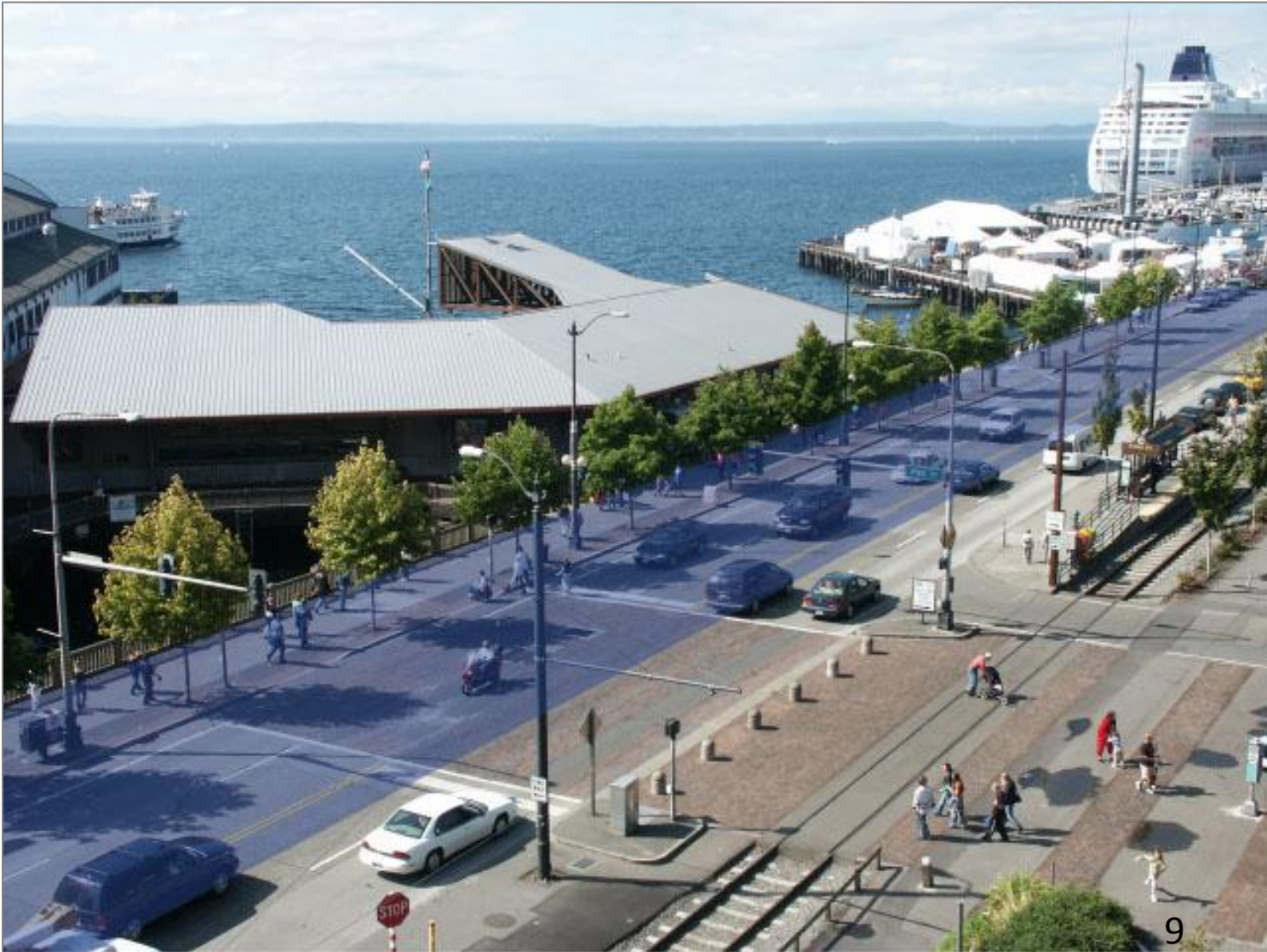
Type A Seawall (Union to Broad)
