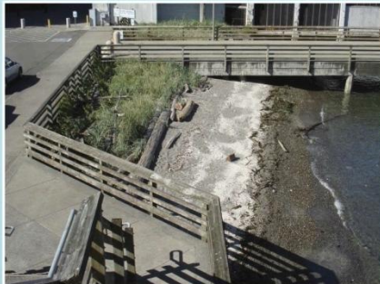
Walkways surrounding beach and habitat bench, Juneau, Alaska. Photo by Peter Levey.
