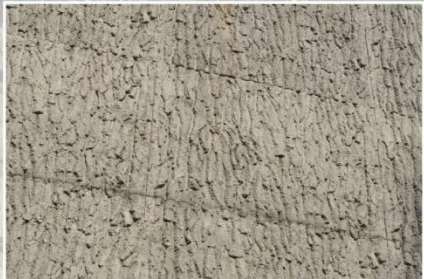
Naturalistic concrete wall texture. Seattle, Washington. Photo by J. A. Brennan Associates.
