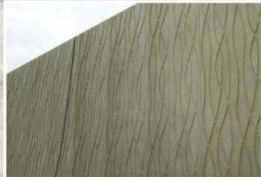
Formlined concrete wave. Photo courtesy of Fitzgerald Formliners.
