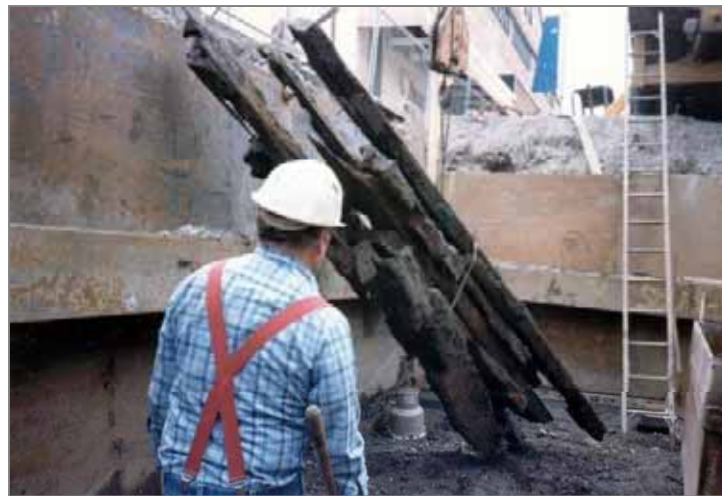
1986 relieving platform repairs (to right)
