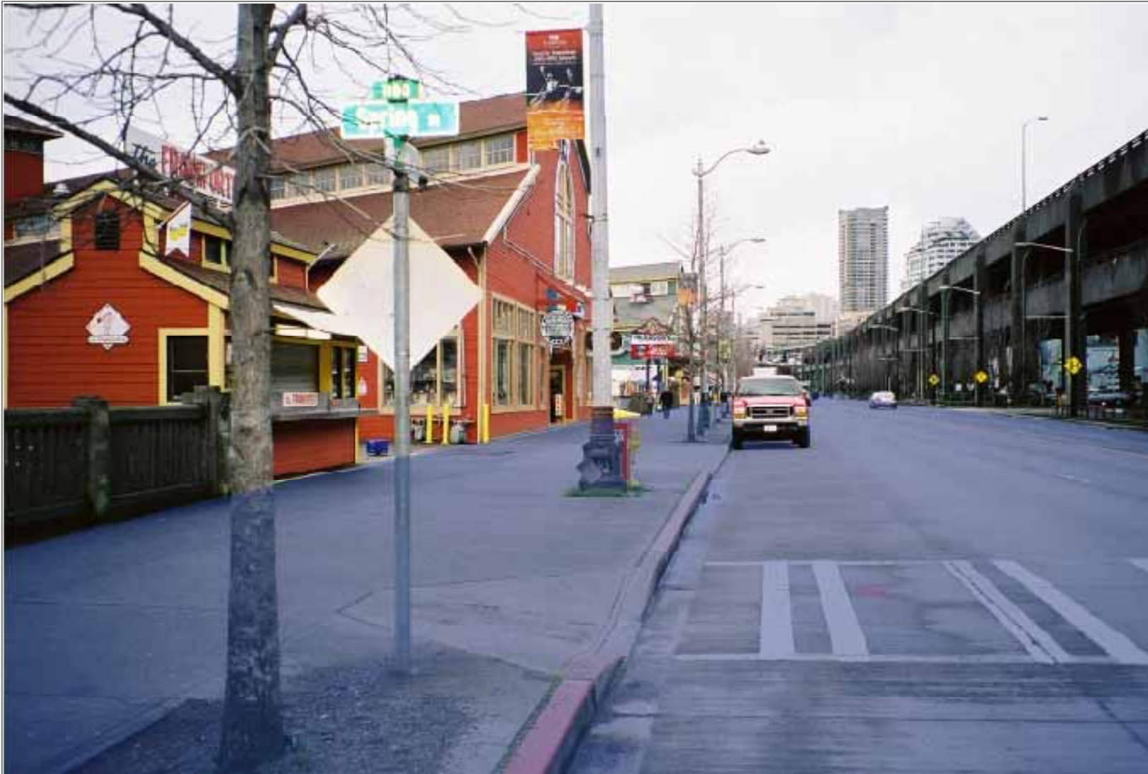
Type B Seawall (Madison to Union)
