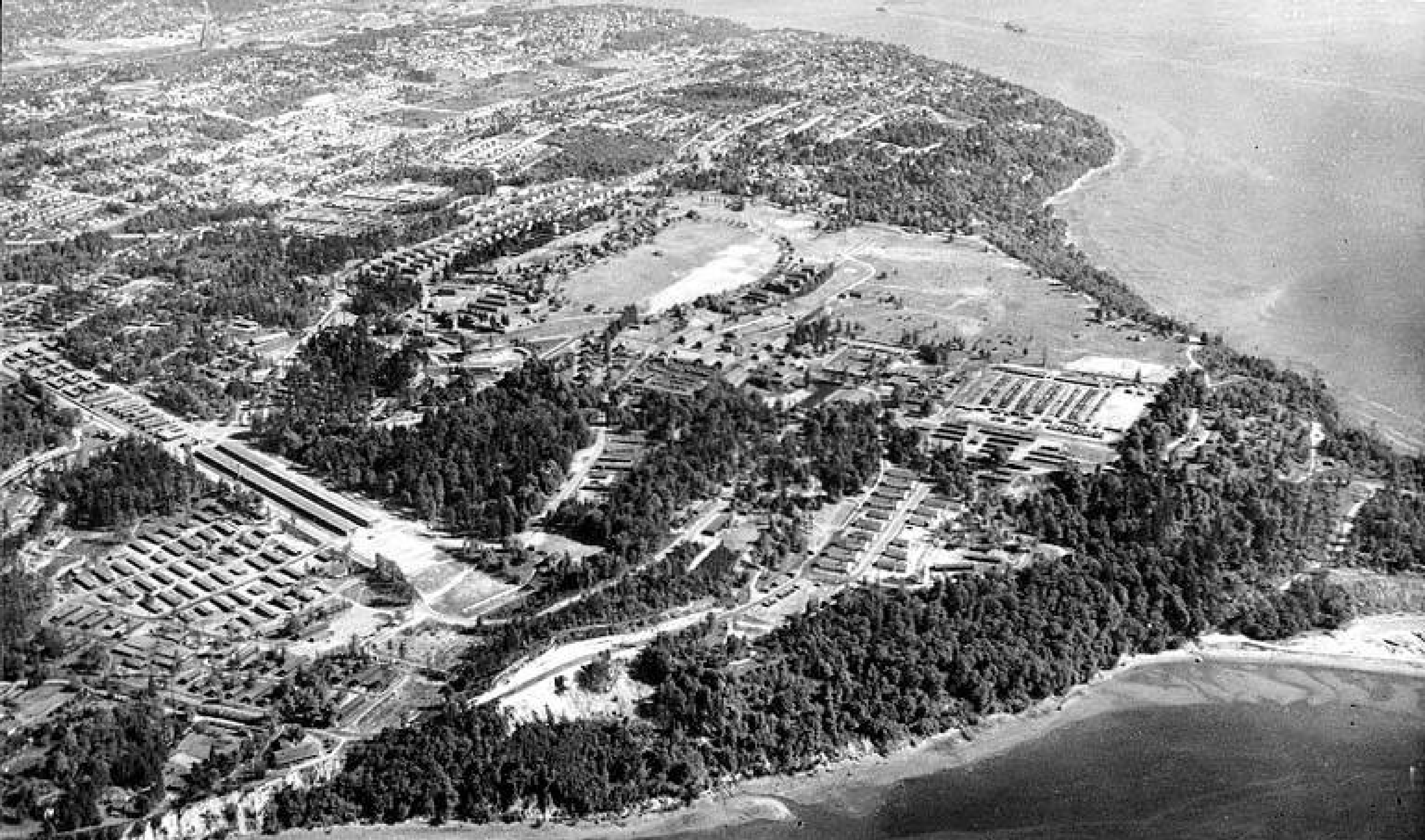
Fort Lawton - Seattle Wash -
