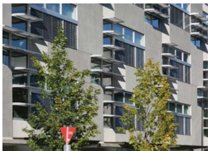
Louvers on the windows help to moderate the amount of sunlight received into this building, as do the deciduous trees.
