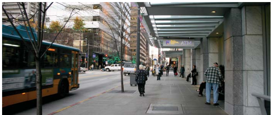
Overhead weather protection and leaning rails have been well integrated into the design of this building, creating a highly comfortable and functional transit zone as well as a handsome streetfront.
