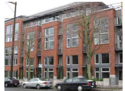
A series of bays and sets of windows lend rhythm and pattern to what would otherwise be a very long, flat façade.
