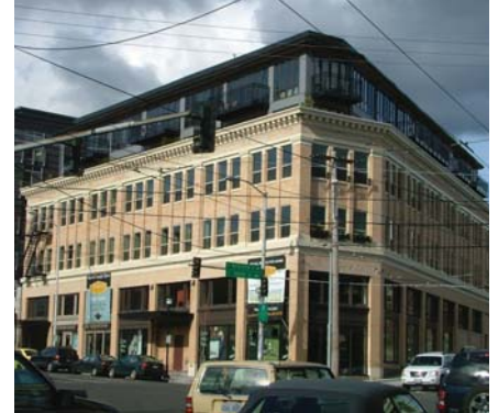
A clear base, middle, and top along with a consistent window pattern lend detail to an otherwise straightforward building form.
