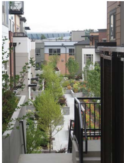
With the building wrapping around all sides of a large block, this project was able to create a large open space with views to and from units and good sun exposure for building residents.
