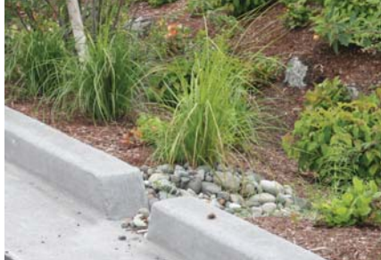
Densely landscaped with native plants, this swale is designed to hold street run-off and release it slowly into the stormwater system.
