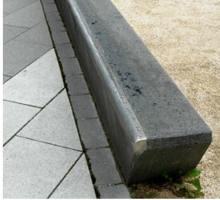
LANDSCAPE CURB WALLS
