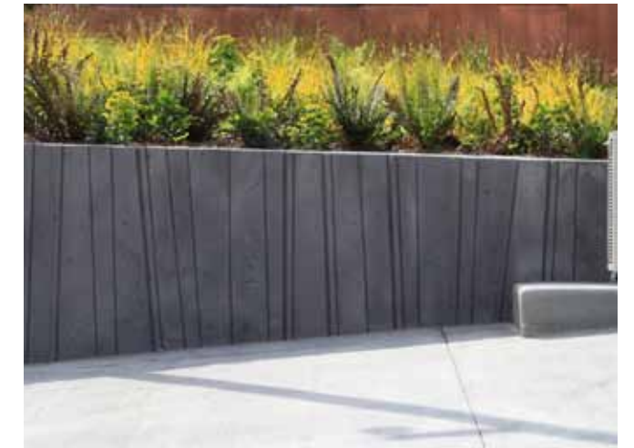
Site walls follow dark-concrete form liner precedent of phase 1
