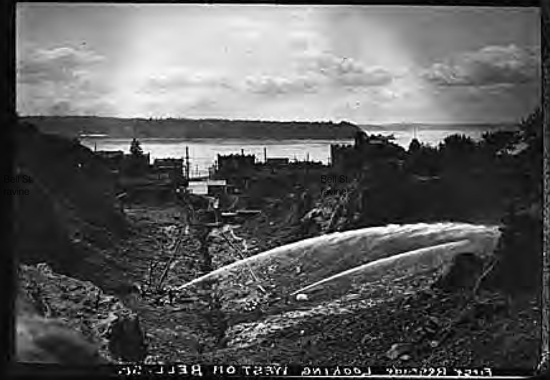
first regrade looking west on bell street
