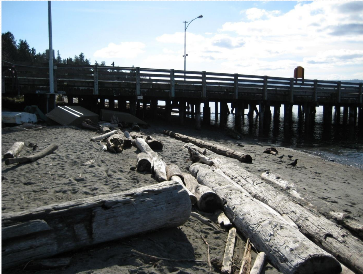
Beach Area Fronting Pump Station (looking south toward ferry terminal)
