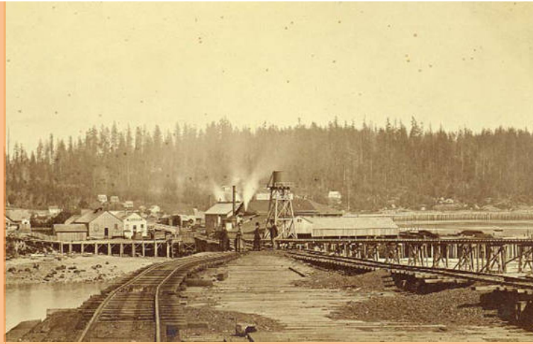
1880 KING ST. COAL WHARF LOOKING EAST
