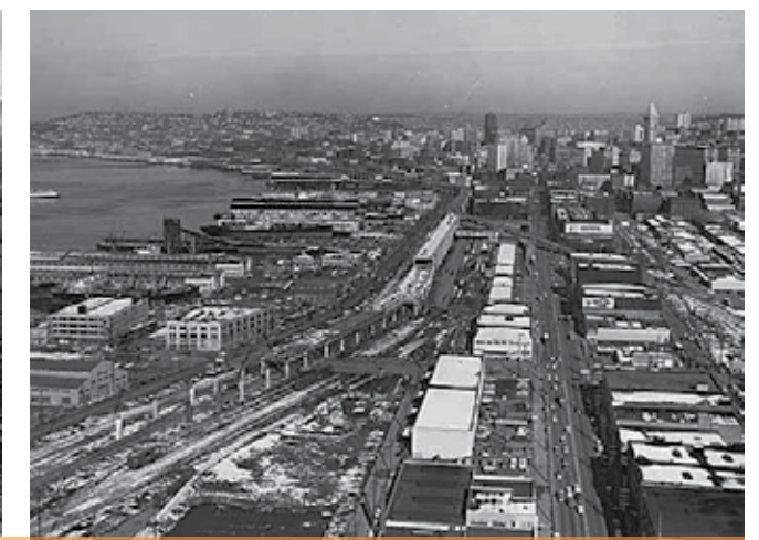
1957 VIEW NORTH OF VIADUCT CONSTRUCTION
