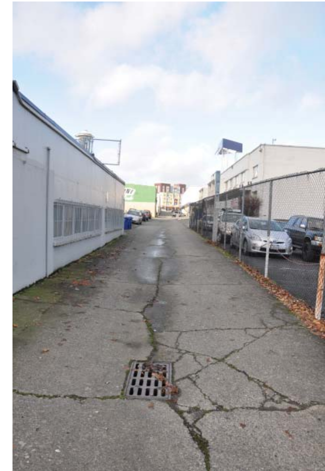
Block 21 Alley (looking North)
