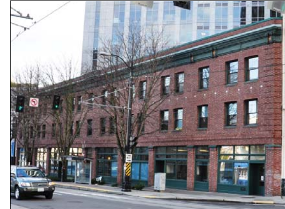
2008 Westlake office building with retail • Human scale • Street front retail
