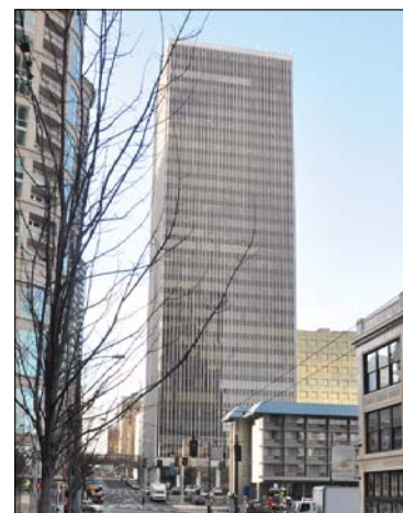
Westin Office Building • Elemental geometry in plan • Glass and metal curtainwall
