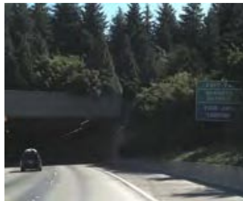
Native northwest on I-90 Mercer Lid
