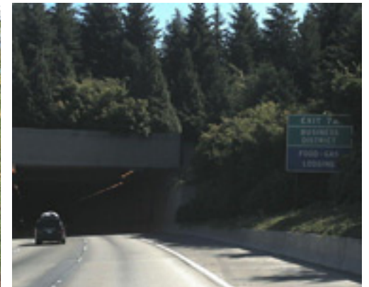
Native northwest on I-90 Mercer Lid
