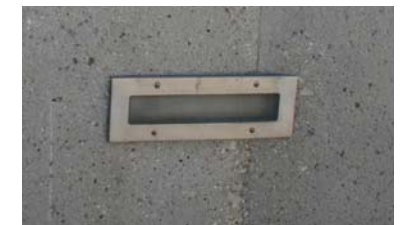
Site lighting in CIP walls
