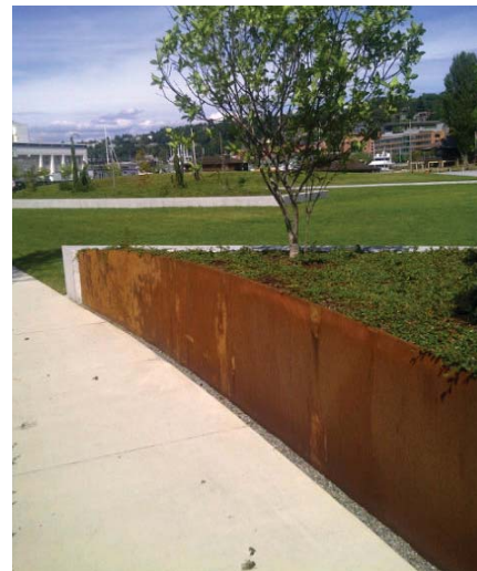
Cor-ten Steel Wall
