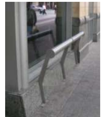
BUS LEAN BARS TYPICAL ALONG BUILDING
