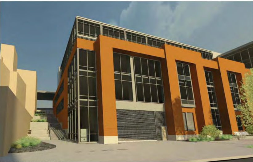
LOOKING EAST AT NORTH STAIR
