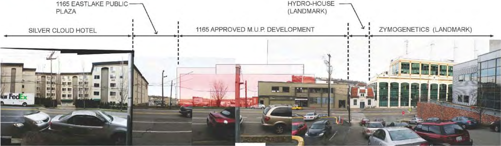
Existing Panorama looking west
