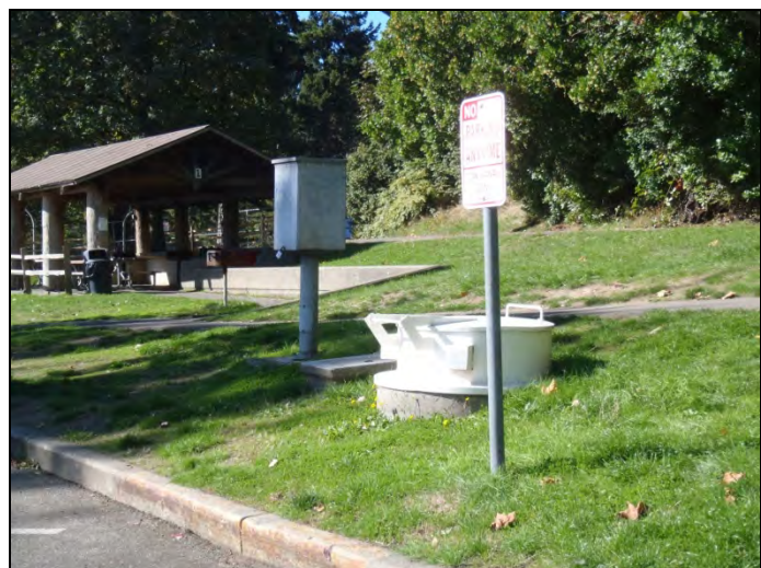
Seattle Parks Sewage Pump Station
