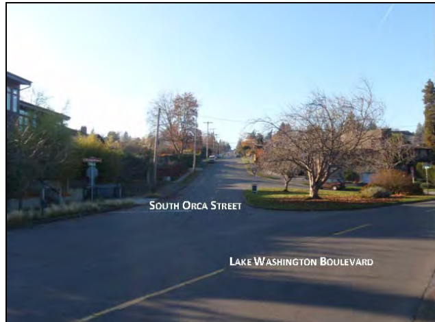
Construction Route 1 Access – looking west
