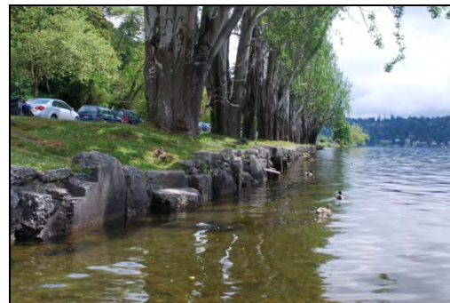
Parking Lot 2 Shoreline Wall
