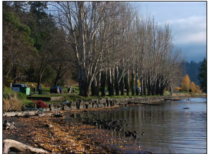
Existing bulkhead near Parking Lot 2
