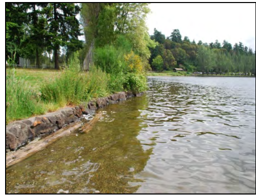
Tennis Court Shoreline Wall
