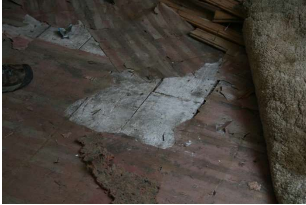
Figure 4 - Flooring materials removed to expose underlying floor joists
