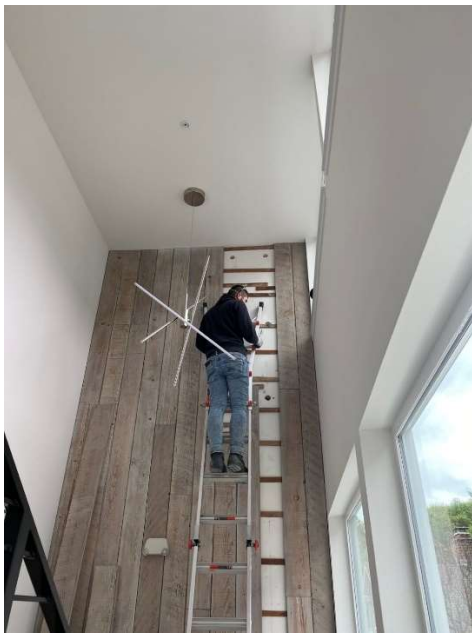
Figure 18 Painted shiplap being installed at Taghus
