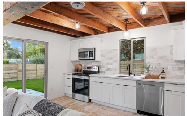
Figure 25 ShipLap product as ceiling joists in third Maple Lane home
