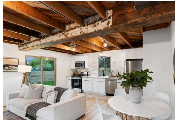
Figure 24 ShipLap product as ceiling joists in second Maple Lane home
