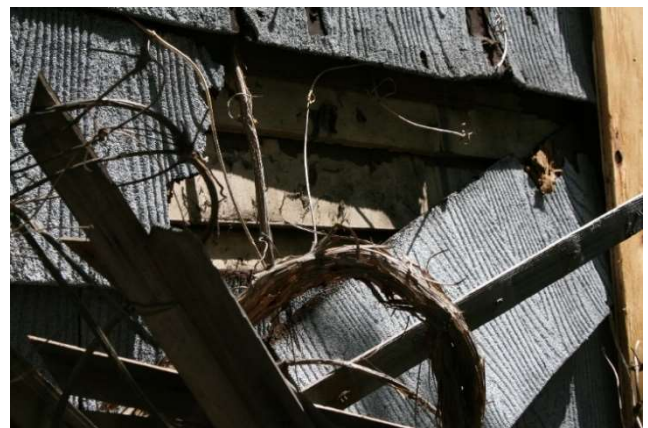
Figure 3 – Newer asphalt siding pulled aside to reveal the original wood siding beneath.
