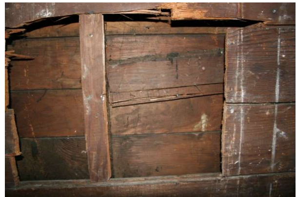
Figure 7 - Cutaway area of top floor showed an additional layer of shiplap
