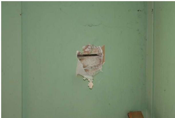
Figure 5 - Dry wall removed revealing lath.
