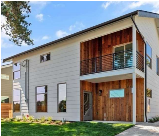
Figure 21 ShipLap product as decorative exterior siding on the homes at Maple Lane
