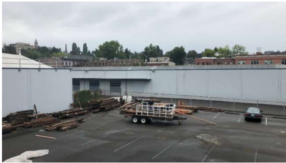
Figure 10 The rear parking area of the Curtain Factor
