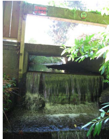
Photo 3: Private driveway crossing with 4.5 ft drop - water feature (photo by OCI)
