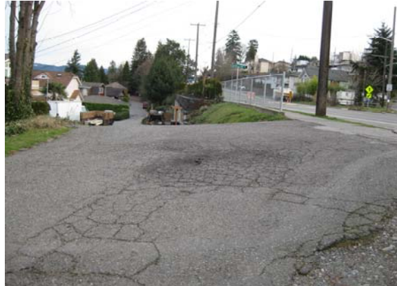
Photo 7: Existing private driveway/access road off of Rainier Avenue S. (photo by OCI)
