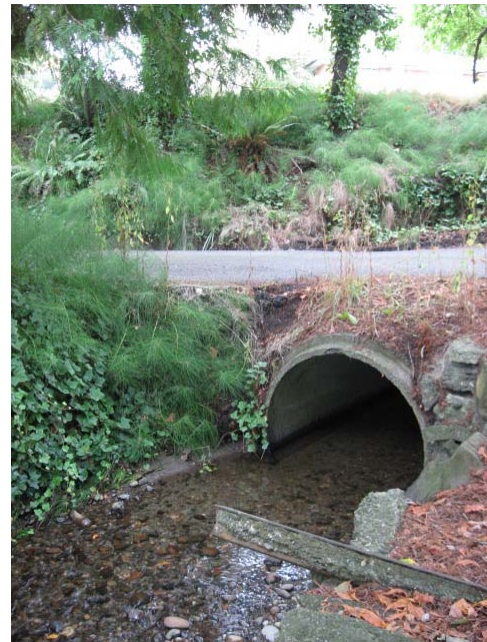
Photo 8: Culvert at private access road, start of Reach 3 (photo by OCI)
