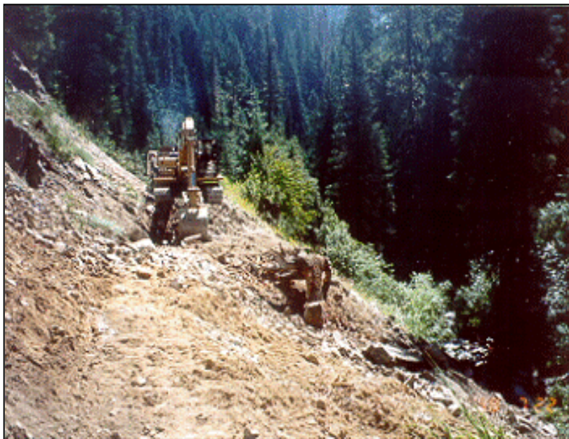
Decommissioning restores natural drainage and stream crossings.
