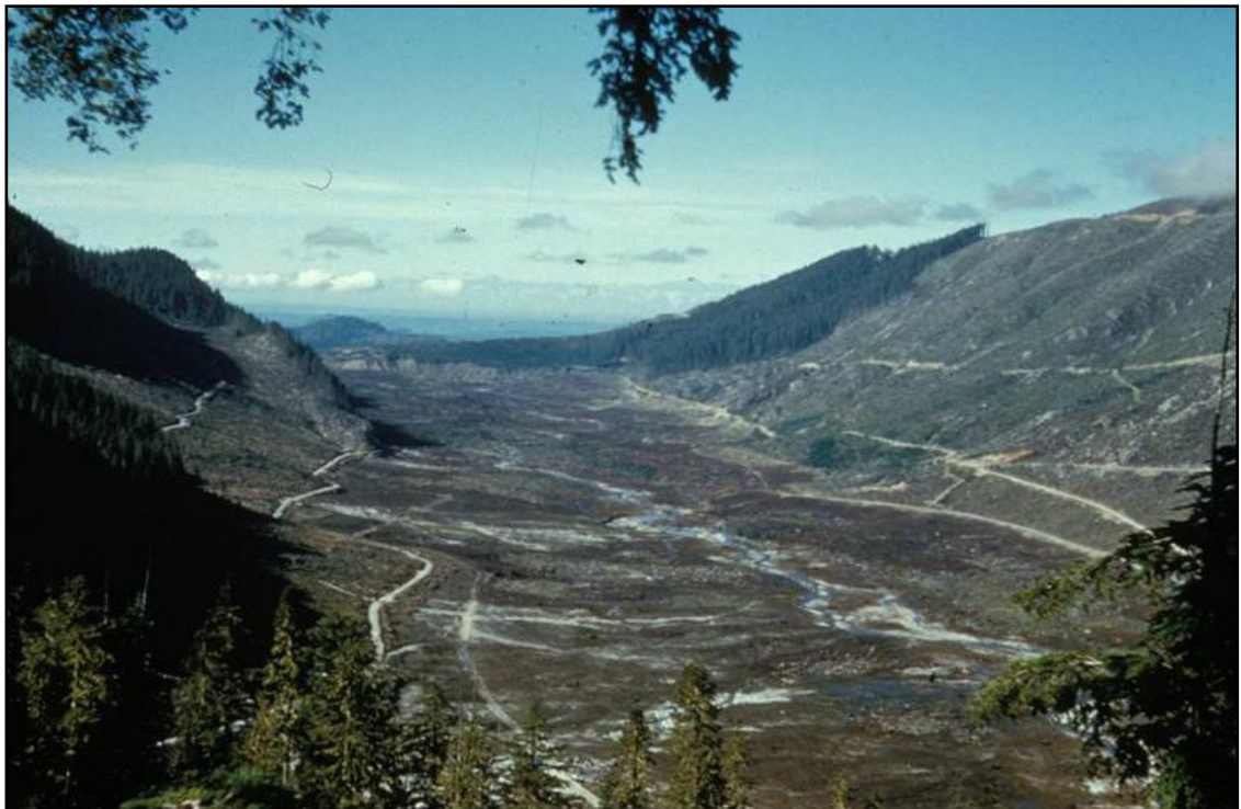
This 1960s photograph shows forest roads on steep valley slopes that trigger landslides.
