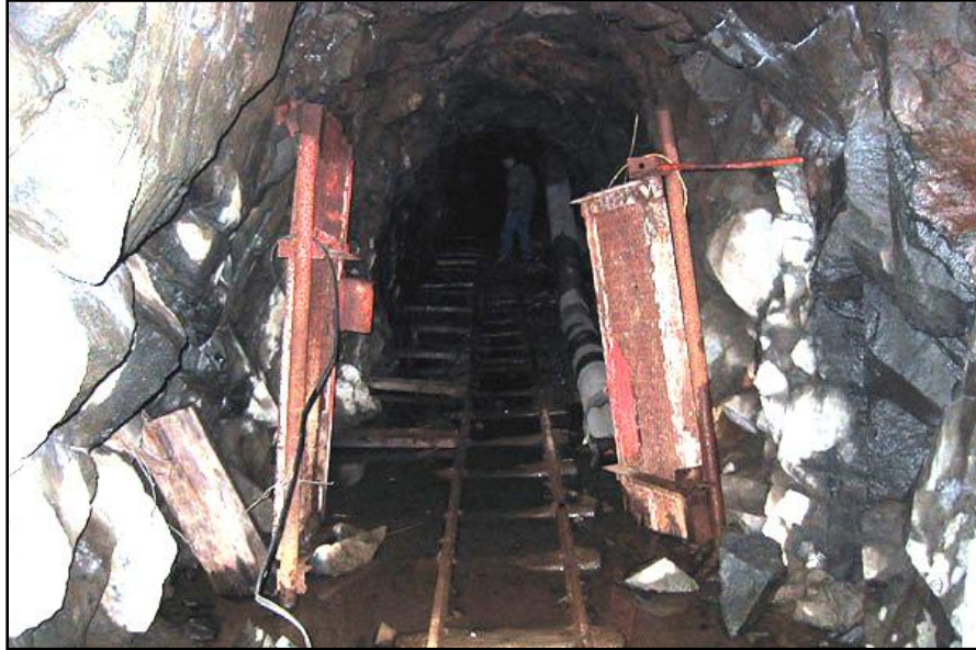
The current gates at Damon Mine are easily pushed aside, making this a popular, and potentially dangerous, destination.
