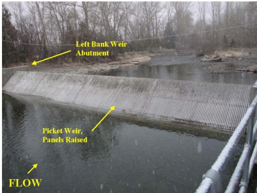
Photograph 2. Picket weir at this fish collection facility on Lostine Creek (Lostine, Oregon) is raised to impede fish passage. Photograph from Bonneville Power Administration. 2013. Lolo Creek Permanent Weir and Fish Trapping Facility Preliminary Environmental Assessment. January.
