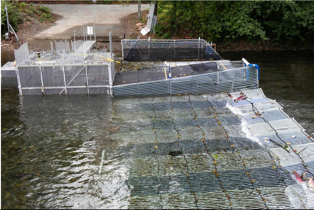
Photograph 1. Picket weir at this fish collection facility is raised to impede fish passage. Location is undetermined.
