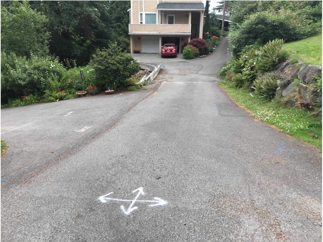
Figure 1. Looking towards the east end of NE 124 th Street, where the new catch basin will be installed.
