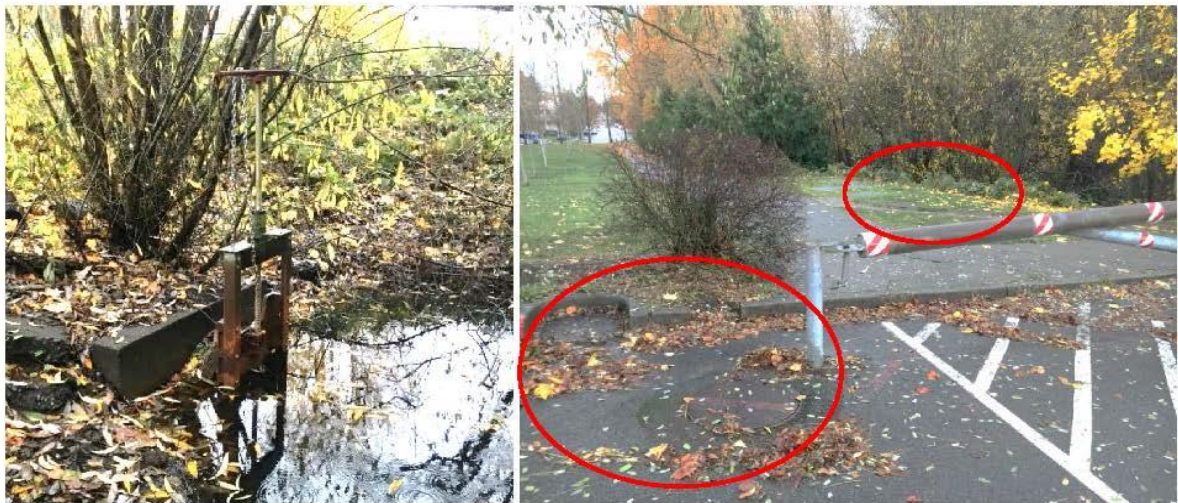
Photo at right shows the view of the underground diversion structure and the oil & water separator locations. Photo at left shows the sluice gate on the 24-inch outfall from the diversion structure
