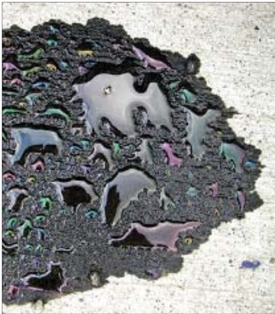
Oil deposits on pavement (photo by Bennett)
