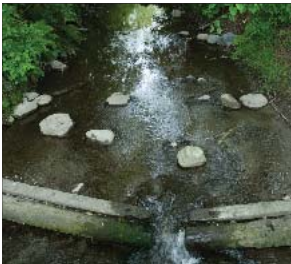
Log deflectors along lower Piper's Creek (photo by Bennett)
