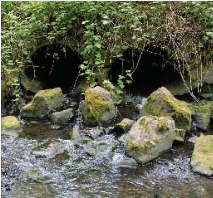
Twin pipes outfall along Piper's Creek (photo by Bennett)
