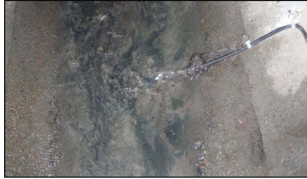
Figure 3-44. LES30_042-205A covered by debris
