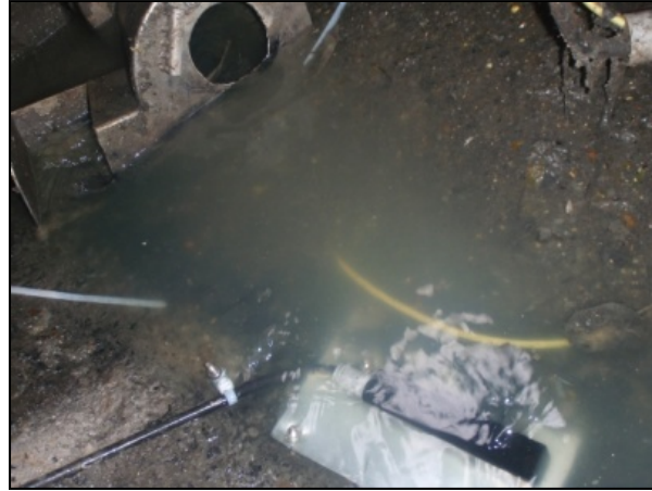
Figure 3-54. LES35_046E-138 HydroBrake cleanout gate open
