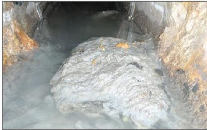
Figure 3-38. Bump upstream of meter at LES026_042-270
