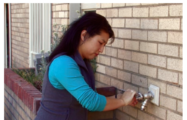
Fixing outdoor leaks is the topic of one of four “Fix a Leak” videos posted on www.savingwater.org .
