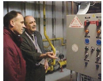
Cornell Amaya of SPU and Tom Nance, Chief Engineer of Group Health Hospital, inspect a new medical air compressor.
