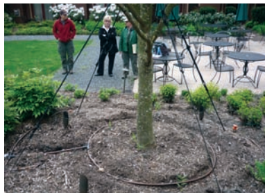
Debbie Rannfeldt of Woodinville Water District views the drip irrigation that replaced a section of in-ground irrigation system at Willows Lodge in Woodinville.
