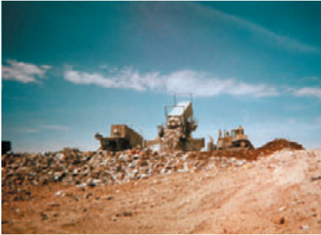
Garbage being dumped from shipping containers at the Columbia Ridge landfill.
