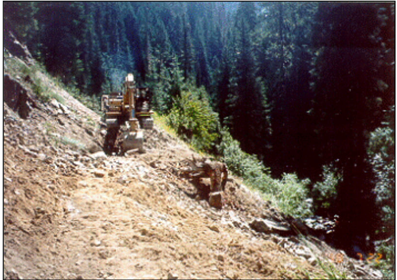
Decommissioning restores natural drainage and stream crossings.
