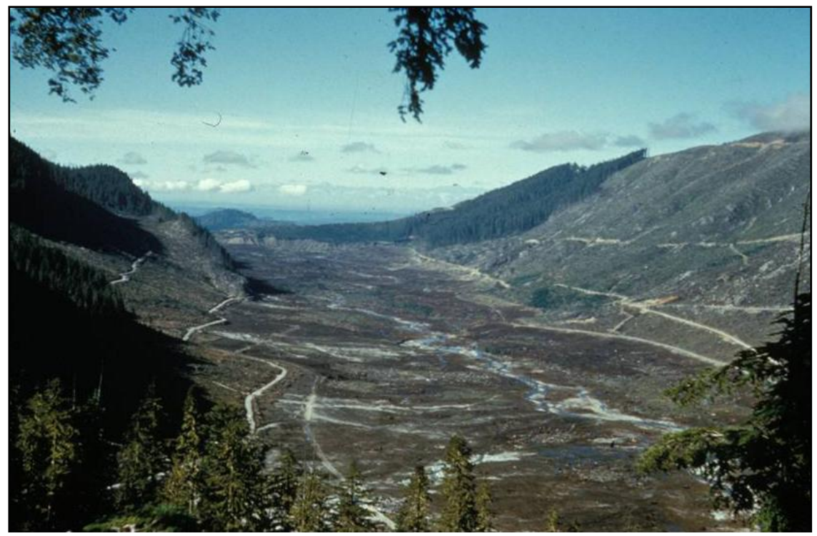
This 1960s photograph shows forest roads on steep valley slopes that trigger landslides.
