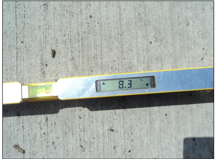
Curb Ramp Running Slope Photo
