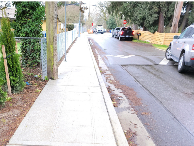
Sidewalk on 37th Ave S for Wing Luke Elementary School
