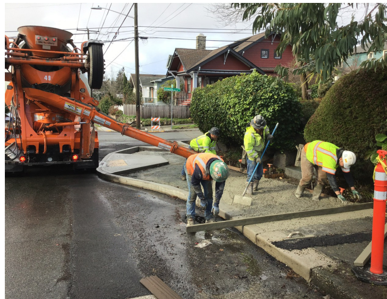
SDOT crews constructing a curb bulb
