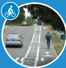
Improved bike lanes for a safe and connected citywide network
