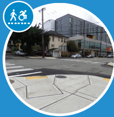
Upgraded crossings for people walking and curb ramps for ADA accessibility
