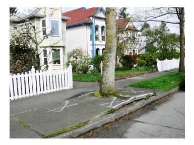
An asphalt shim is used to keep the sidewalk functioning and safer for pedestrians.
