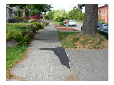
Maximum slope is 1:4 For temporary sidewalk shims and grinding.
