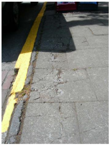
Tree root heave created by too little growing space. By increasing the size of the tree pit, the sidewalk and the growing conditions are improved.
