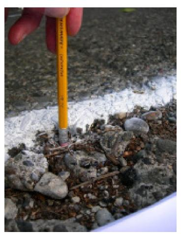
Holes and cracking in the sidewalk can vary in size and must be filled.
