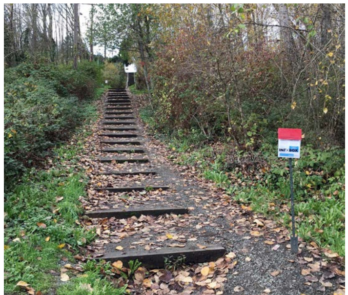
Existing stairway at S Hanford St between Cheasty Blvd S and Morse Ave S
