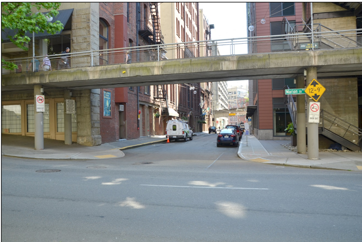
Figure 18. Post Avenue Bridge, view to the south; note Marion Street Overpass in foreground.
