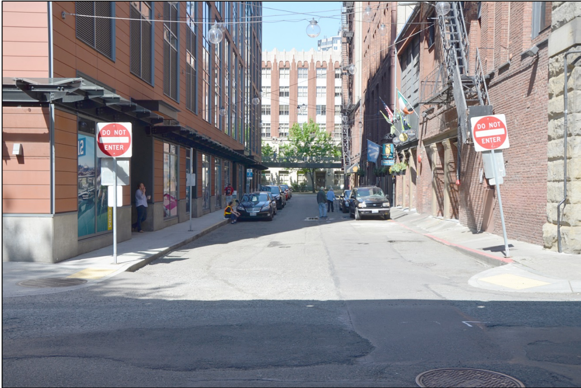
Figure 17. Post Avenue Bridge, view to the north.
