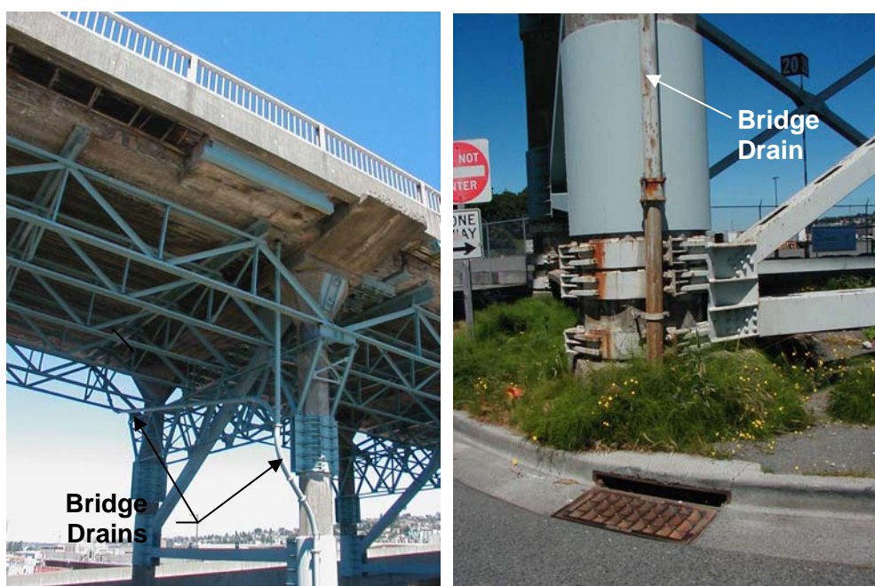
Figure 13 Existing Bridge Drains
