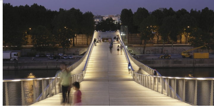
Lighting mounted on handrail
