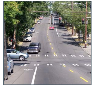
Climbing lanes have been installed on E Union Street to allow slower bicyclists riding uphill to be in a bicycle lane and encourage faster bicyclists riding downhill to move further from parked cars and share the travel lane.
