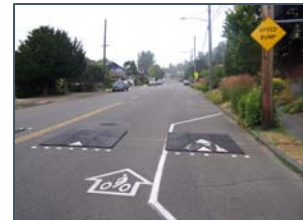
Speed cushions are used on Beach Drive SW to slow traffic on this popular bicycle route.
