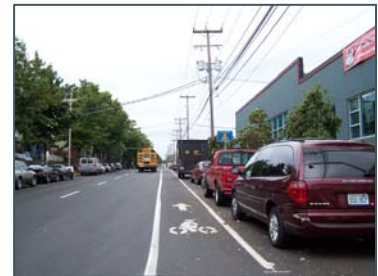
A bicycle lane was striped on Roy Street when the roadway was repaved.
