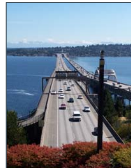
The I-90 bridge trail was constructed as part of the bridge project. A similar trail will be provided on the SR-520 Bridge when it is replaced..
