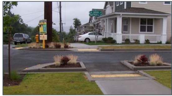
Curb extensions were constructed on SW Juneau Street to slow motor vehicles.
