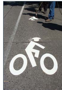
SDOT field crew installs a bicycle lane marking.
