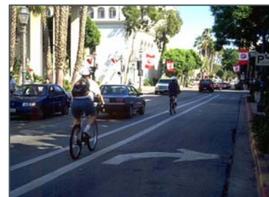
Pocket Lane Stripping, Berkeley, California
