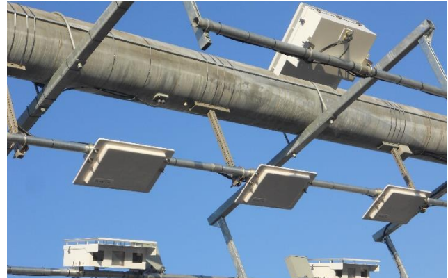
Figure 14 Example of AVI antennas to read transponders and cameras to capture license plates
