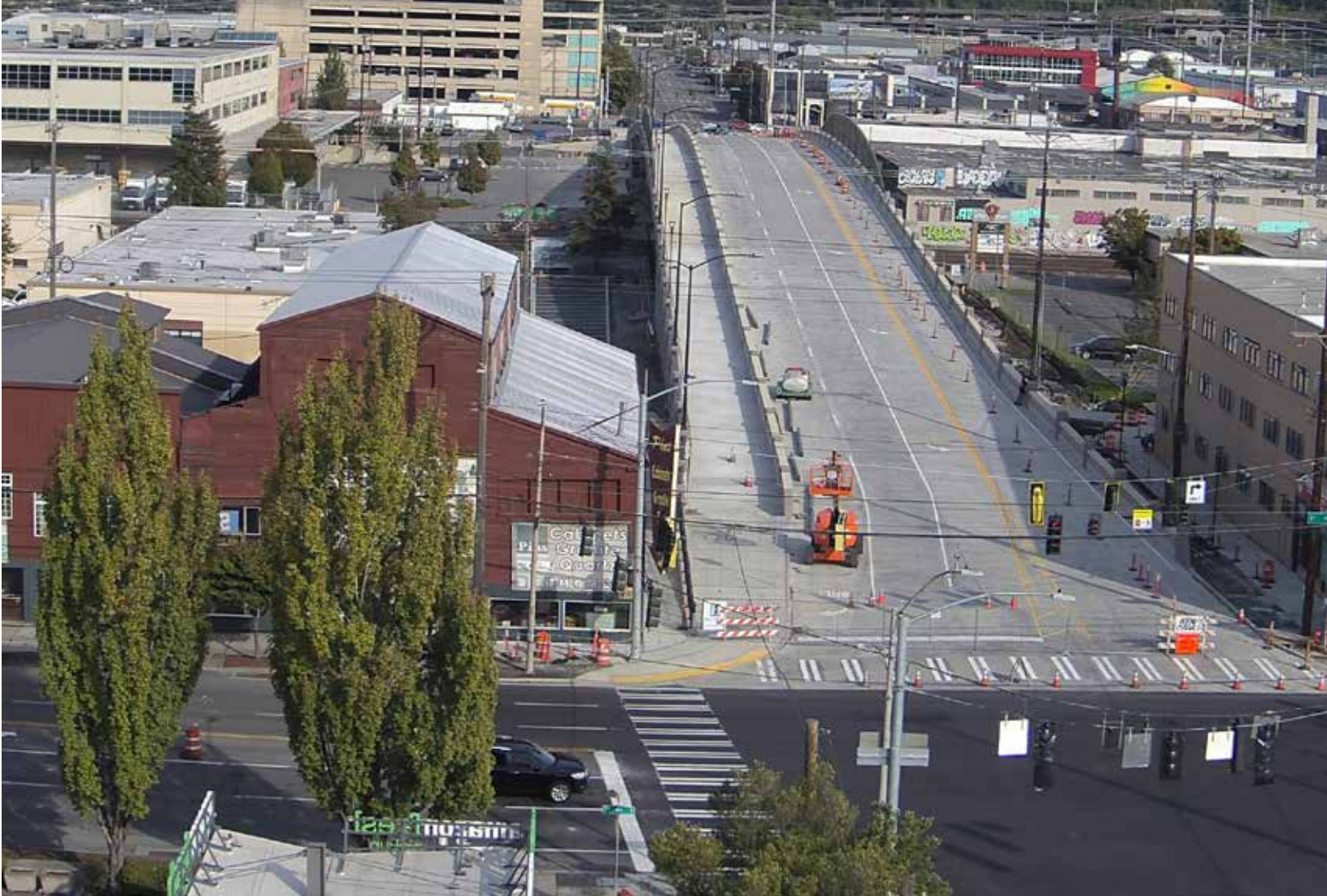
Fall 2020, Lander Bridge Overpass
