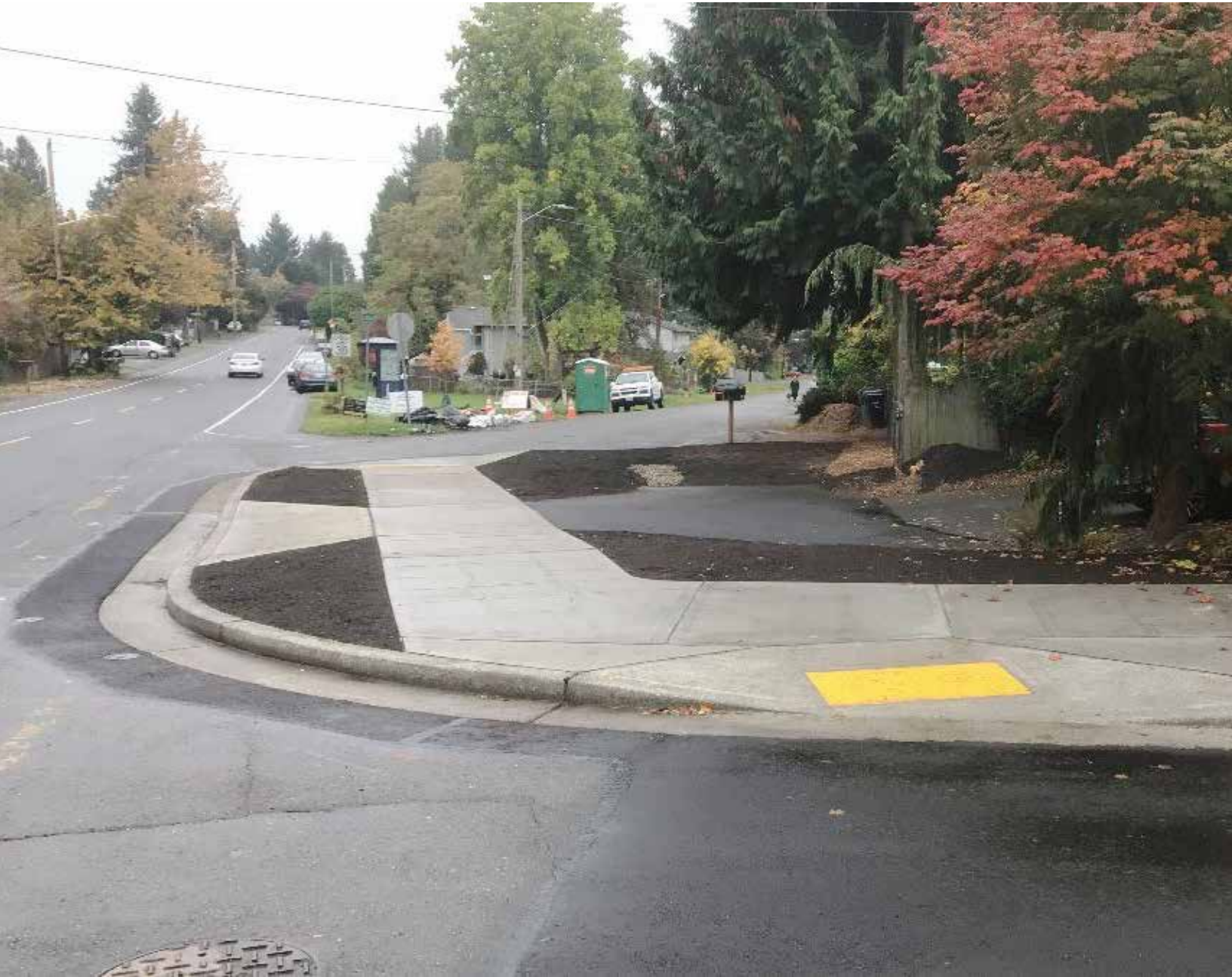
Fall 2019, completed curb bulb
