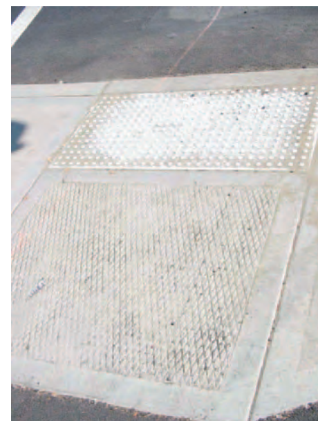
Truncated domes are an important wayfinding tool for visually impaired walkers
