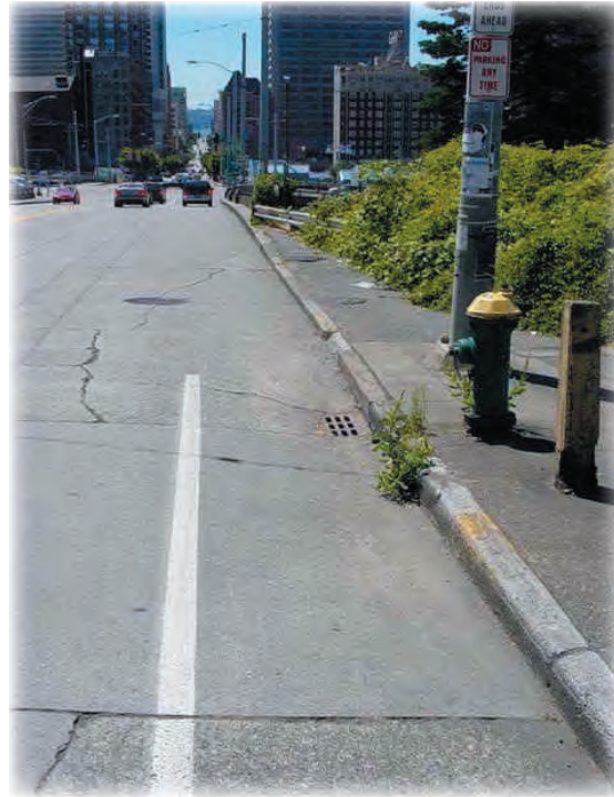
Bike lane and sidewalk end heading southwest on Pine over I-5
