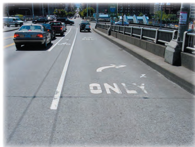
Resumption of southbound bike lane on Pine before Boren
